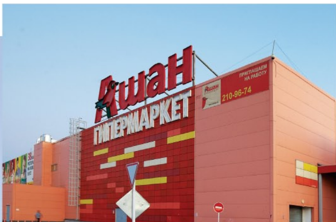
The analog addressable fire alarm system and intrusion alarm system for Auchan hypermarkets in Russia, one of the largest international retail chains
