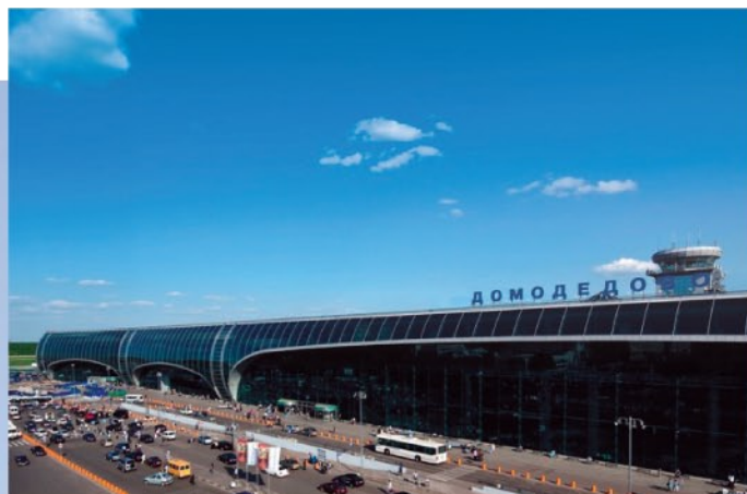
The analog addressable fire alarm system and intrusion alarm system for a group of administrative buildings of Moscow Domodedovo Airport
