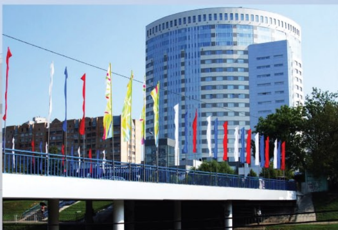
The analog addressable fire alarm system, intrusion alarm system, and access control system for Kutuzoff Tower in Moscow, a class "A" prestigious business center
