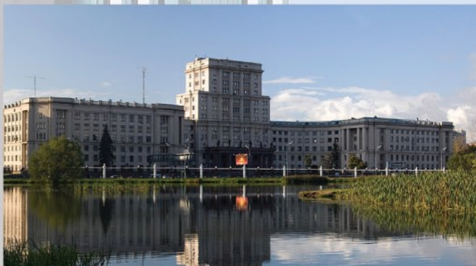
The analog addressable fire alarm system, fixed gaseous extinguishing system, fixed water extinguishing system, access control system for Bauman Moscow State Technical University, the first and one of the largest technical universities in Russia, scientific center and particularly valuable object of cultural heritage of the peoples of Russia
